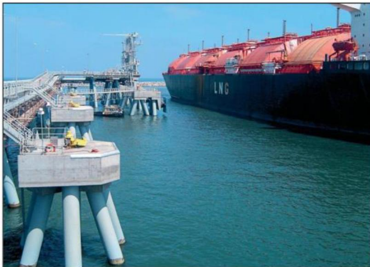
Figure 11: An example of a trestle jetty.
